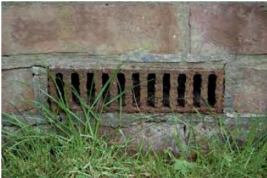
This pic & below: Air bricks on the exterior of the house feed directly into the void under floorboards making the downstairs one of the coldest parts of the house
